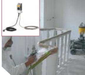
The warmth in the heating hose constantly keeps the coating materials at the ideal working temperature.
